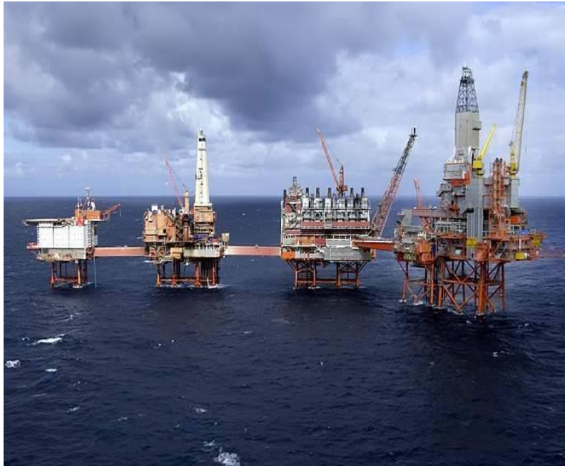
Figure 1: The existing Valhall complex.
