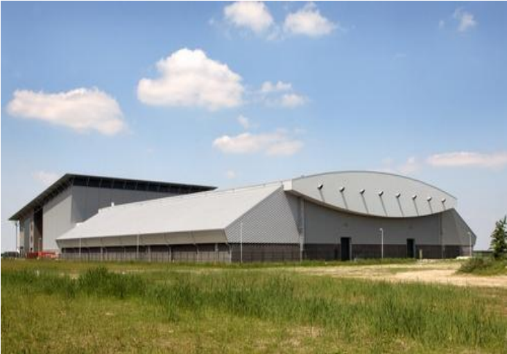
Figure 2 Eemshaven converter station
